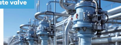
Ultratork multi-turn actuator is suitable for automatic control of gate valves. The independent actuator can output a maximum torque of 1000Nm. Actuator with gearbox can provide even greater output torque.
